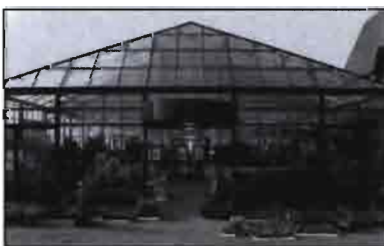
Vista exterior Garden Center.
