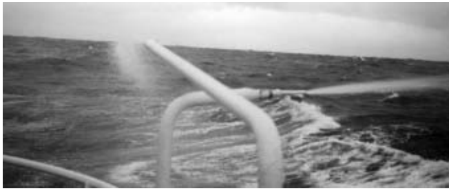
FIG. 2. TWIN WATER CANNONS.
